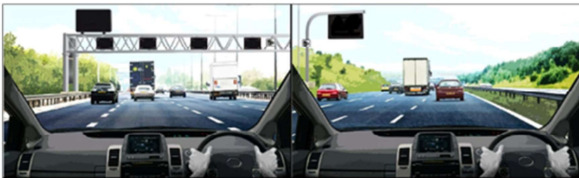
Figure 4139 Blank signals in normal traffic conditions
